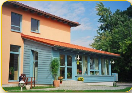
view of building - outer entry area
