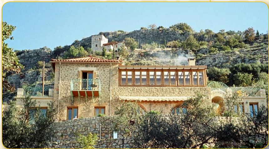
front view of the building
